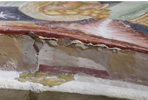
Figure 2. Detail of the damages on the wall paintings caused by the earthquake.
