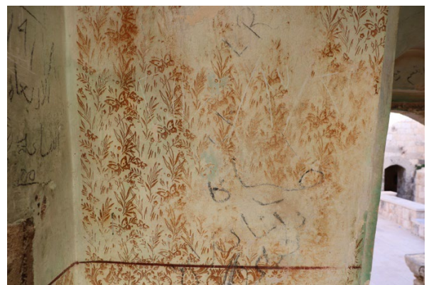
Figure 4. Decorative Pattern applied probably using a stencil roll at the lower thickness of the four arches supporting the dome at Dar ee Abd-Allah, Kur. Salameh, M. (2017, December 31). Dar Abd-Allah (KR_A) [Context Photo].
