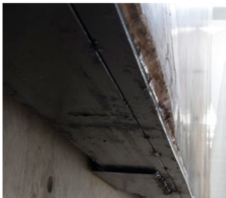
Figure 2. Detail taken in raking light of the damage caused by the detachment of the wall painting.
