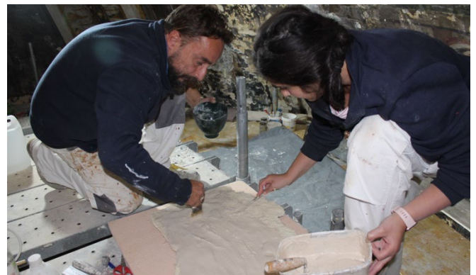
Figure 4. Applying a thick grout on the back of the reinforced.
